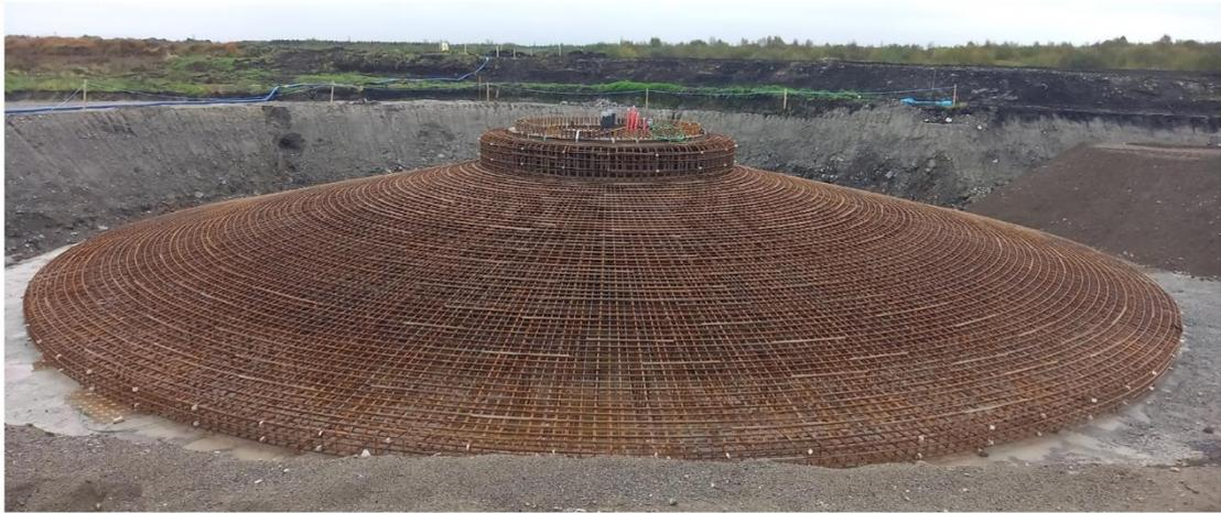
Plate 4-2 Turbine Base Anchor Cage
