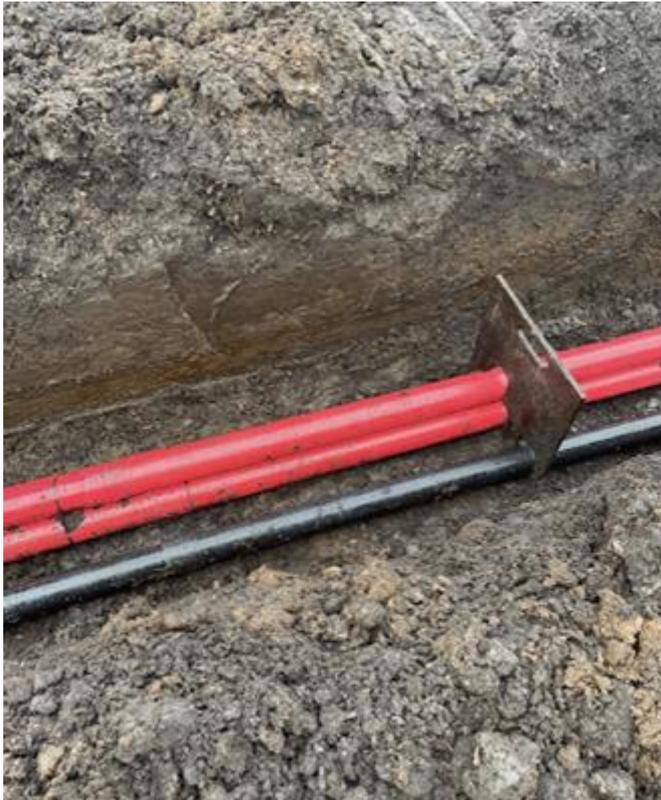
Plate 4-10 Typical Cable Trench View left, reinstated trench, right. Source Bord na Móna.
