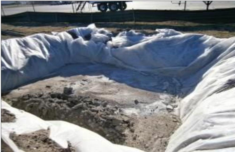
Plate 4-5 Concrete Wash Out Area
