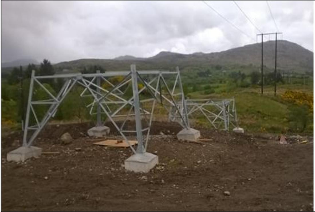
Plate 4-12 Steel lattice tower foundation complete
