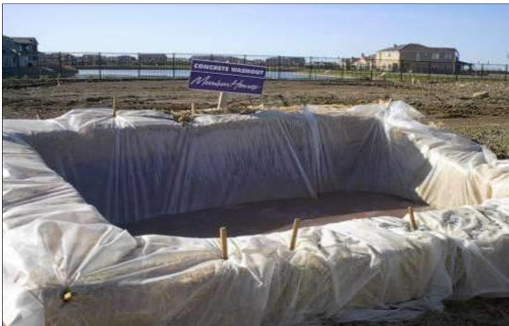
Plate 4-4 Concrete washout area
