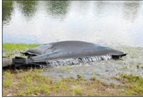
Plate 4-7 Silt bag under inspection
