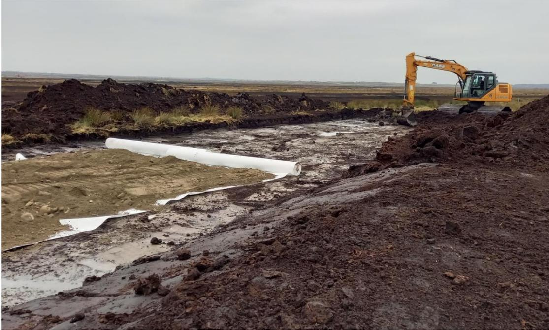
Plate 4-9 Internal road under construction demonstrating laying of geogrid/geotextile. Source Bord na Móna.
