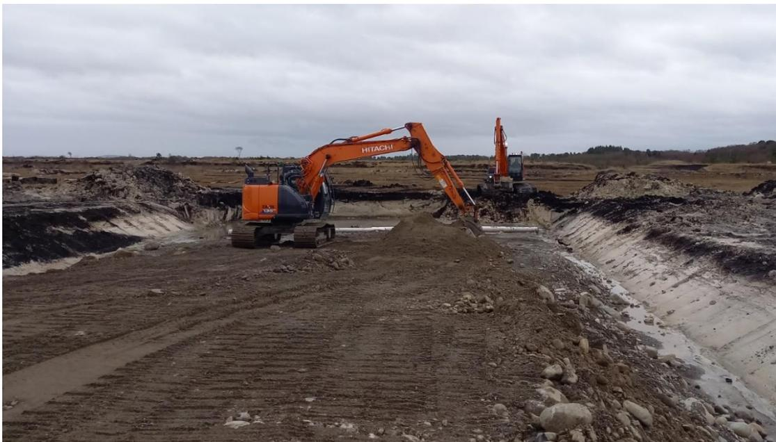
Plate 4-8 Internal roads under construction using the excavate and replace method. Source Bord na Móna.
