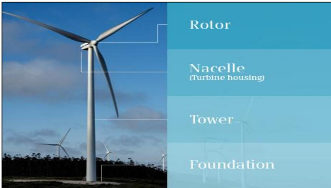
Plate 4-1 Wind Turbine Components
