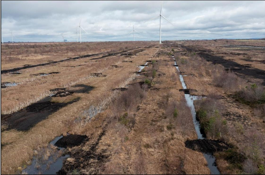
*Photo 2-3: Peat dams installed on cutover bog within the Clonreen windfarm site*
