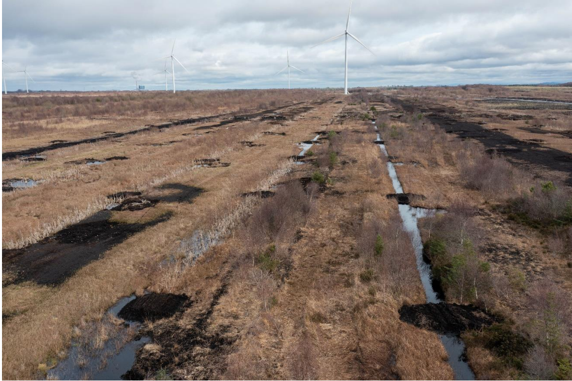
Plate 10-1 PCAS peatland rehabilitation implemented in the form of drain blocking proximal to wind farm infrastructure at the Clonreen Wind Farm Site.
