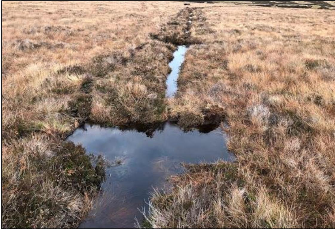
*Plate 2-2. Example of peat dams to be used for on-site drain blocking. This will re-establish and maintain a hydrological regime for the required peatland rehabilitation.*
